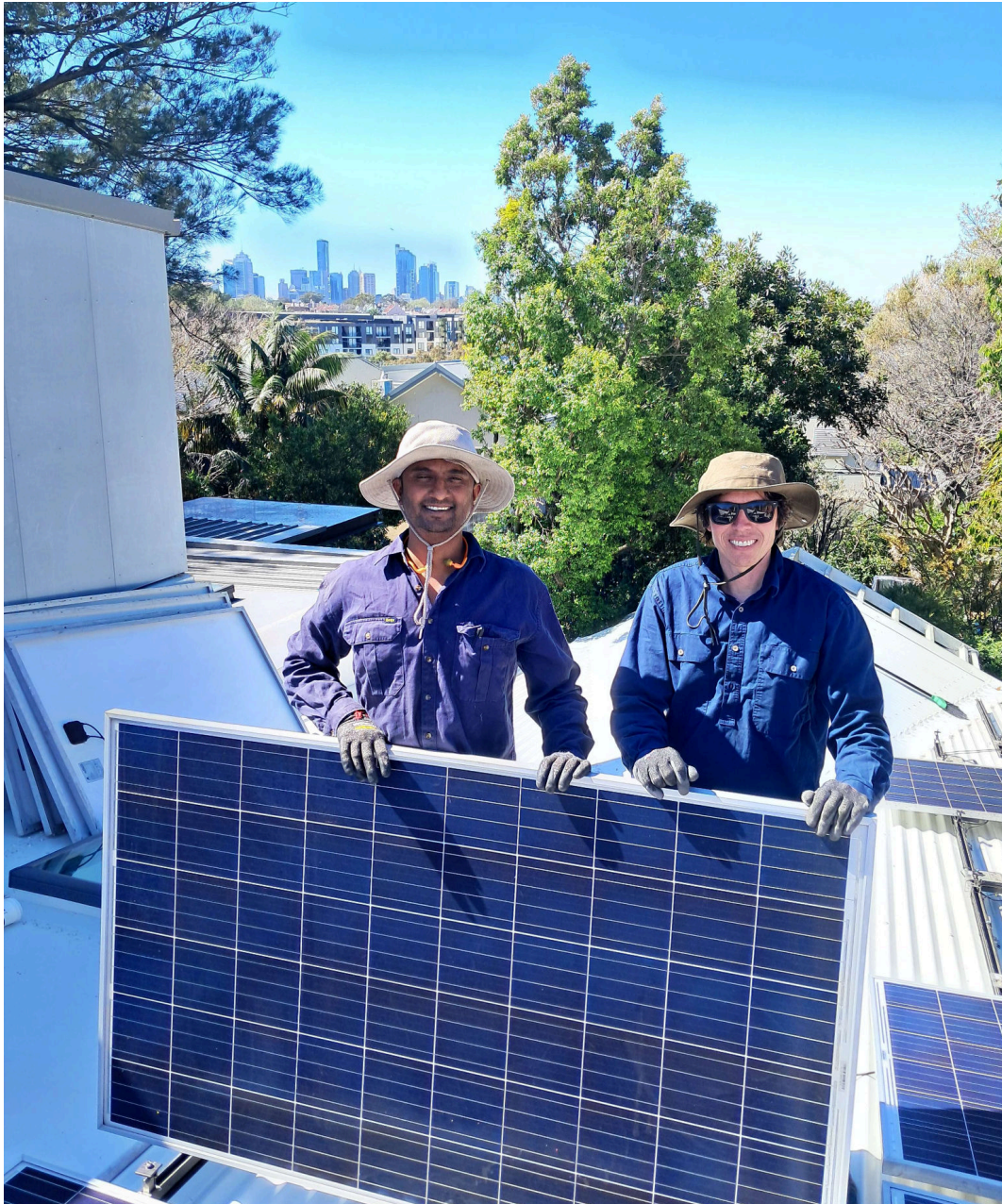
Installers Neil and Tillman on a sunny Inner West rooftop.
