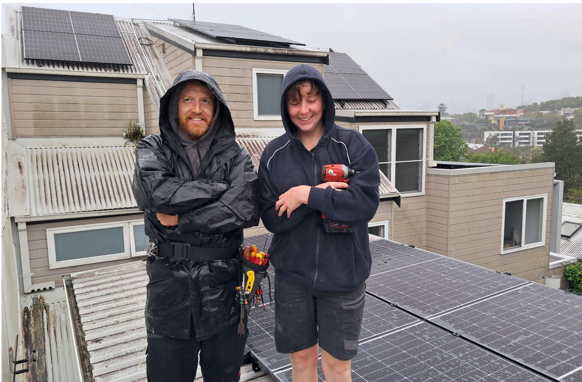
Installers Mick and Jess braving a rainy day.
