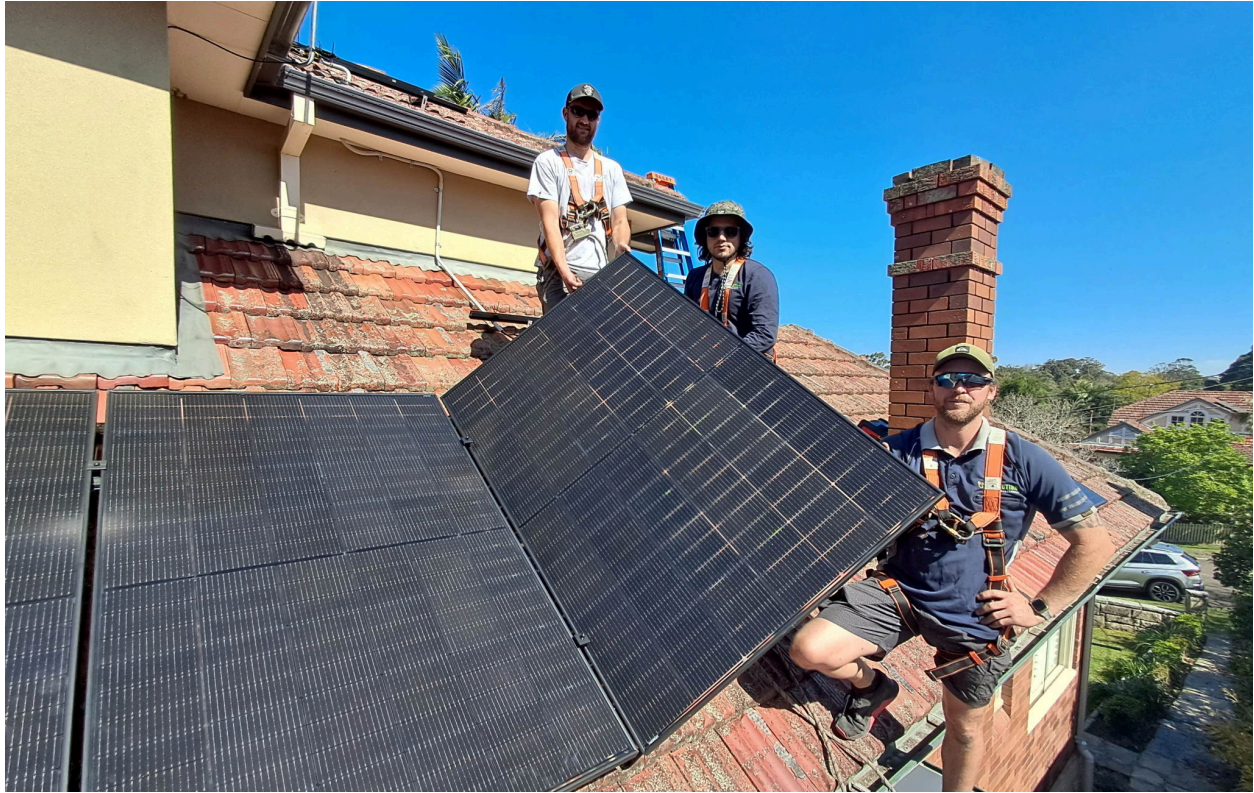
Installer team Zac, Pablo, and Phil on a sunny terracotta roof.
