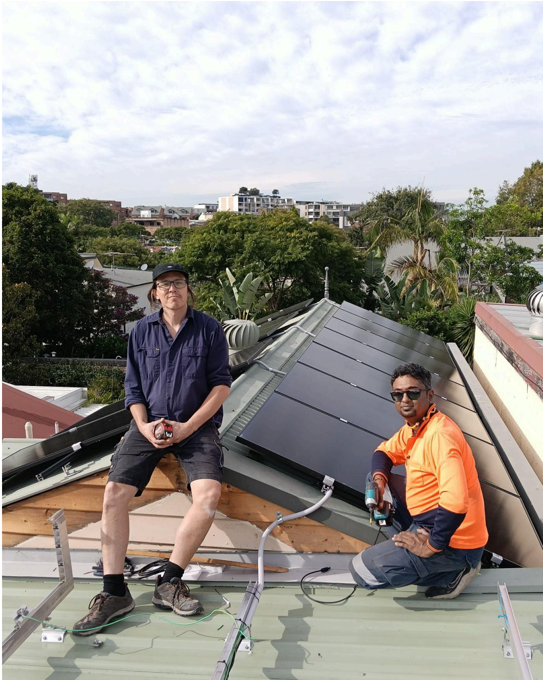
Installers Tillman Kiesow and Nafneel Prasad partway through installing a new solar system on a sunny Inner West rooftop.
